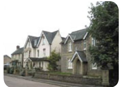
Nos 4 to 8 Fairfield's Road
